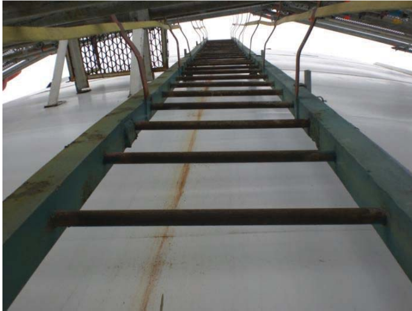
Pic 35: Vertical ladder, slightly misaligned.
