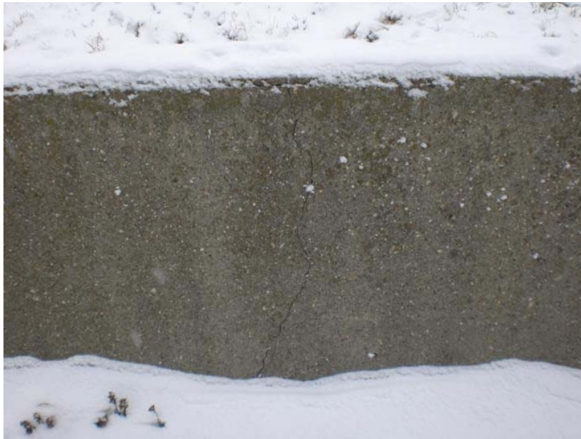
Pic 4: Crack in dike wall over whole height.
