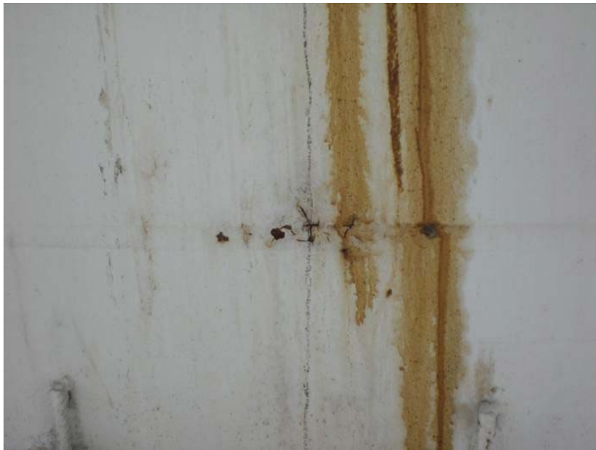
Pic 38: Product stains, paint failure, corrosion.
