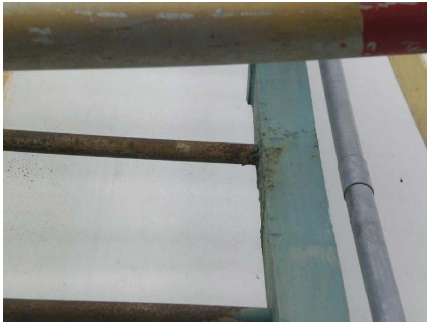
Pic 36: Corroded rung connection.
