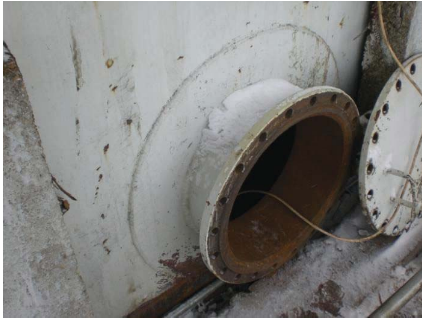
Pic 17: Manhole. No telltale hole present in the reinforcement plate.
