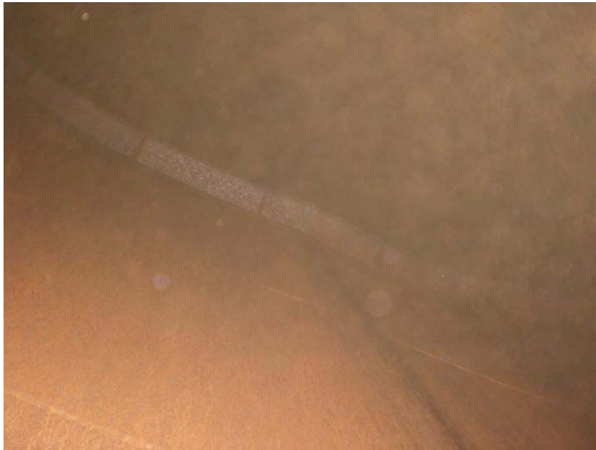
Pic 58: Shell and wind girder deformation in the vicinity of the vertical shell weld.
