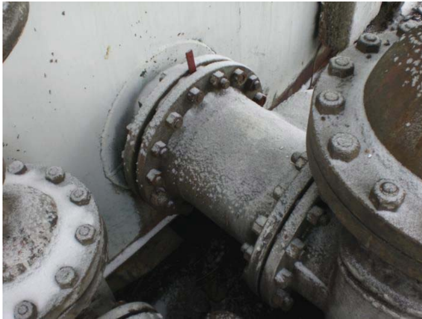
Pic 20: Reinforcement plate made of two halves.
