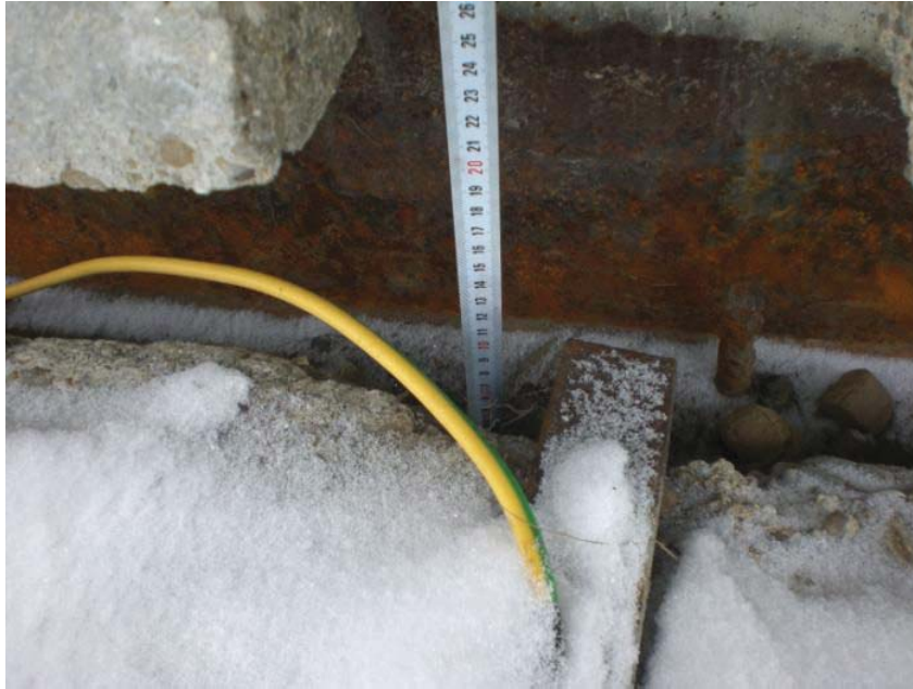
Pic 31: Grounding strap, about 80 mm settlement.
