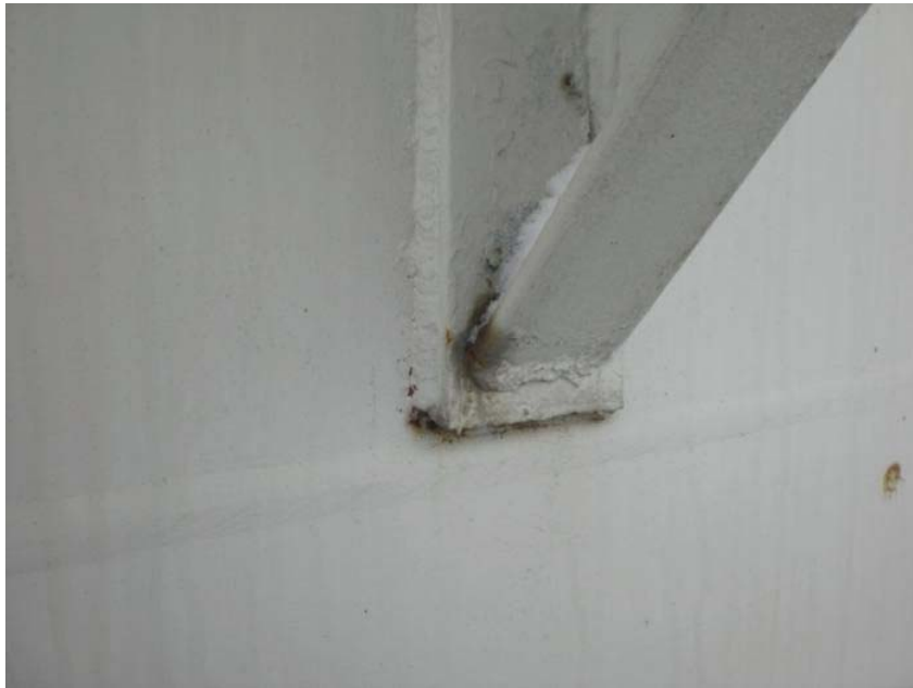
Pic 34: Support for spiral stairway, lack of weld space.
