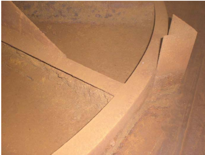
Pic 48: Lateral fixation for center column.
