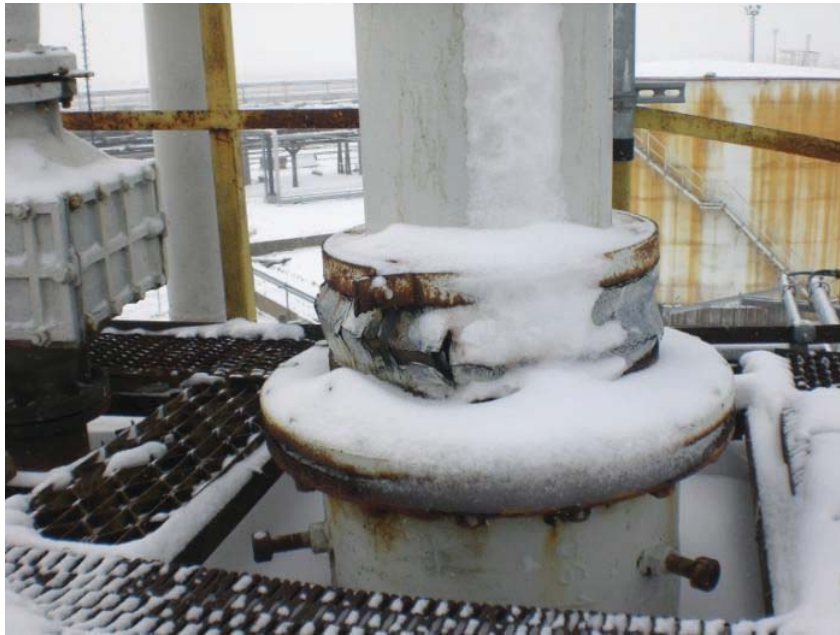
Pic 44: ATG (Radar) connection damaged.
