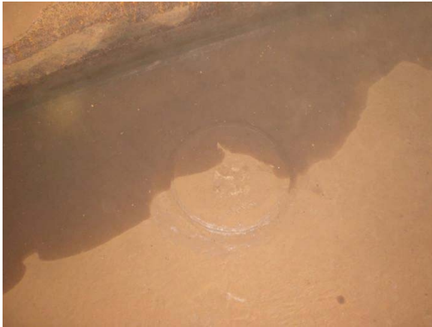
Pic 55: Patch plate or abandoned striker plate.
