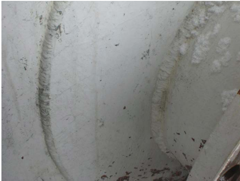
Pic 18: Satisfactory weld work on the manhole.
