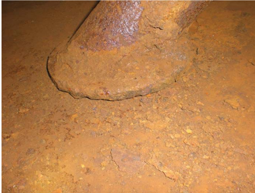
Pic 51: Swivel support pads not seal welded to the bottom plate.
