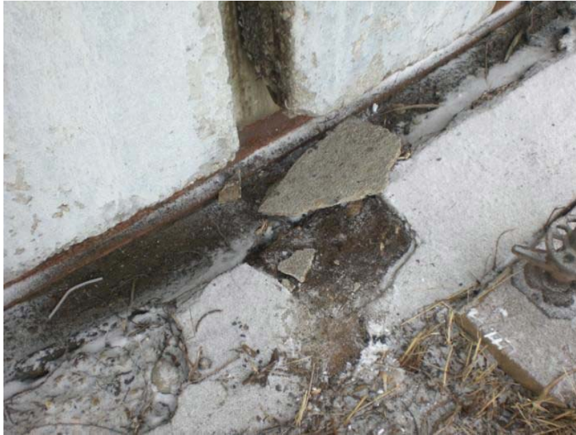
Pic 25: Damaged concrete ring, big gap between concrete ring and tank bottom projection.
