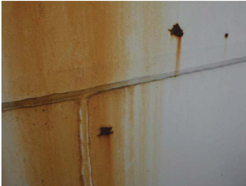
Pic 37: Paint failure, corrosion and product stains on the shell. Origin of staining is the roof, however exact location unknown.
