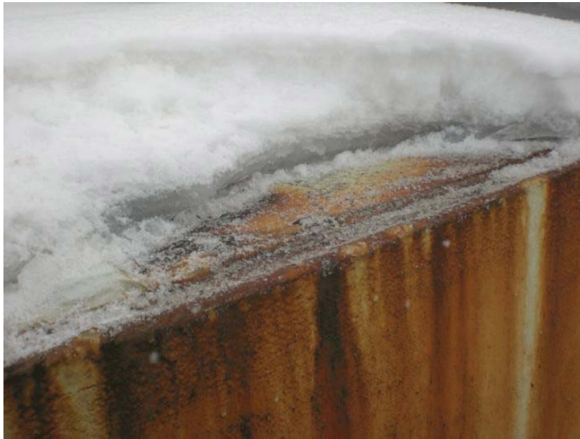
Pic 41: Roof to shell connection. No Top Curb Angle (TCA) present.
