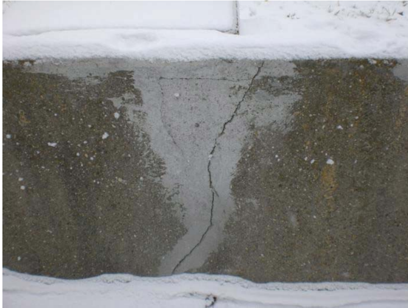
Pic 5: Previously repaired (?) crack in the dike wall.
