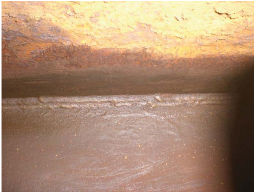
Pic 62: Poor weld work of the corner weld.
