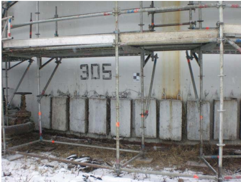
Pic 22: Concrete blocks hanging all over the tank circumference.
