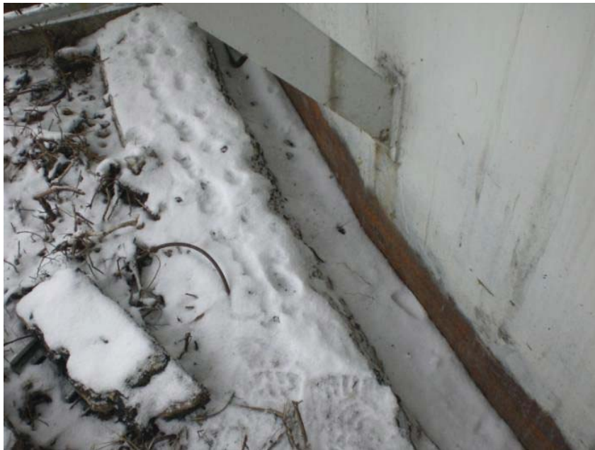
Pic 28: Tank settled about 70 mm into the foundation.
