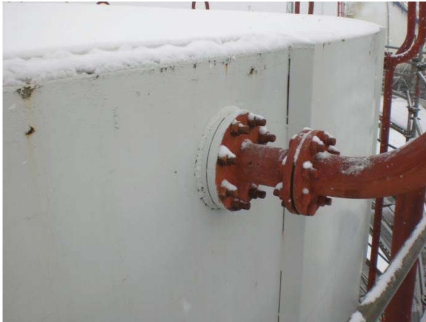
Pic 46: Fire line connection
