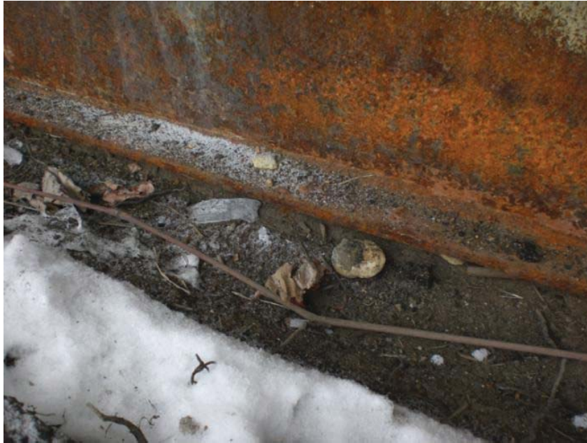
Pic 27: Foundation close up. Bottom projection in fair condition, however soil washed out and gravel visible.
