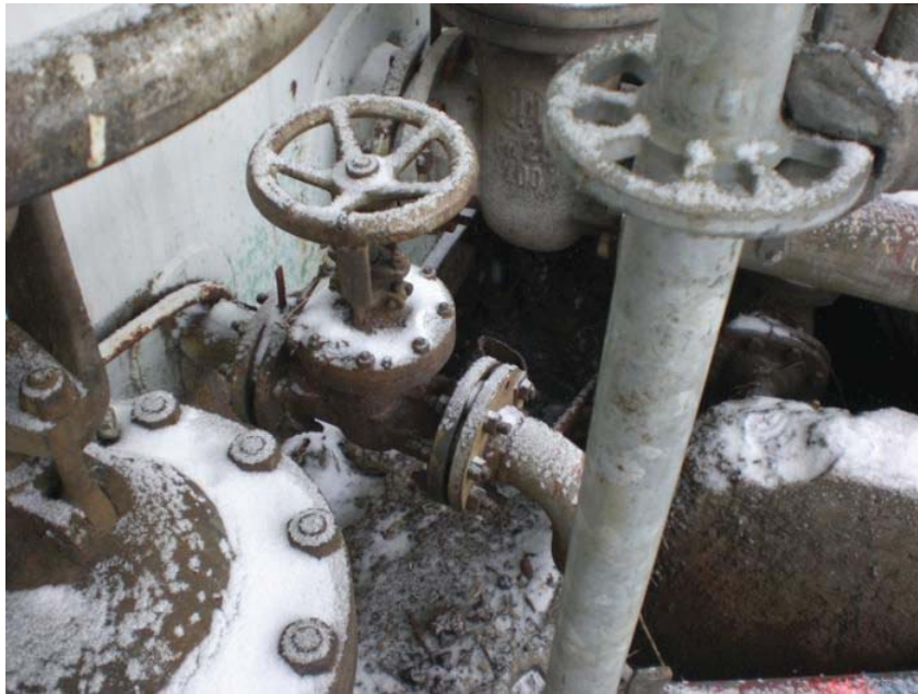
Pic 16: Pipe work, purpose of the pit is unknown.
