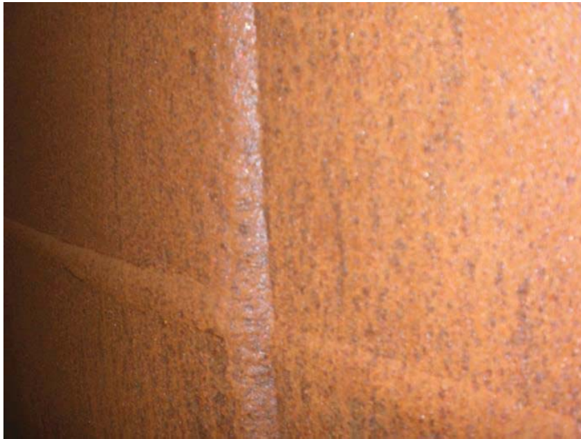
Pic 56: Vertical shell lap weld.
