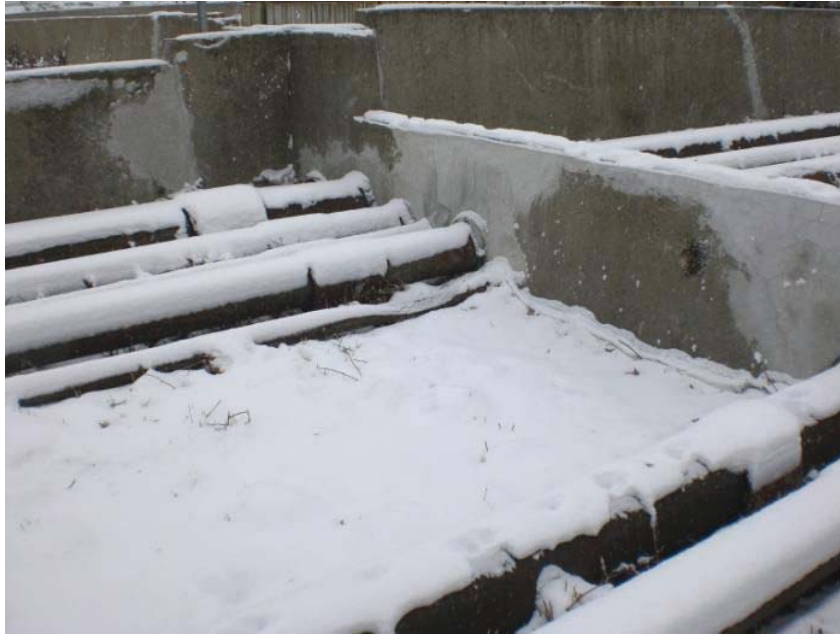
Pic 7: Pipe work in the diked area. Pipes are running through metal sleeves and are surrounded by heavy vegetation.
