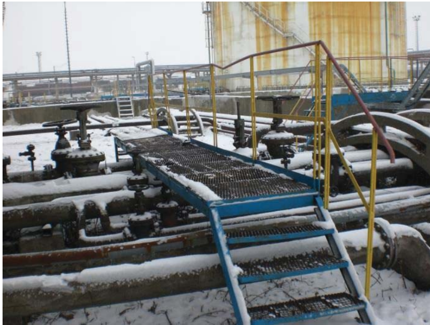
Pic 11: Misaligned, corroded and distorted bridge over pipe work. Handrail facing the tank missing.
