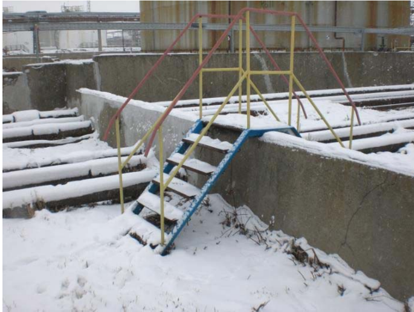
Pic 3: Access Structure, crack in dike wall.
