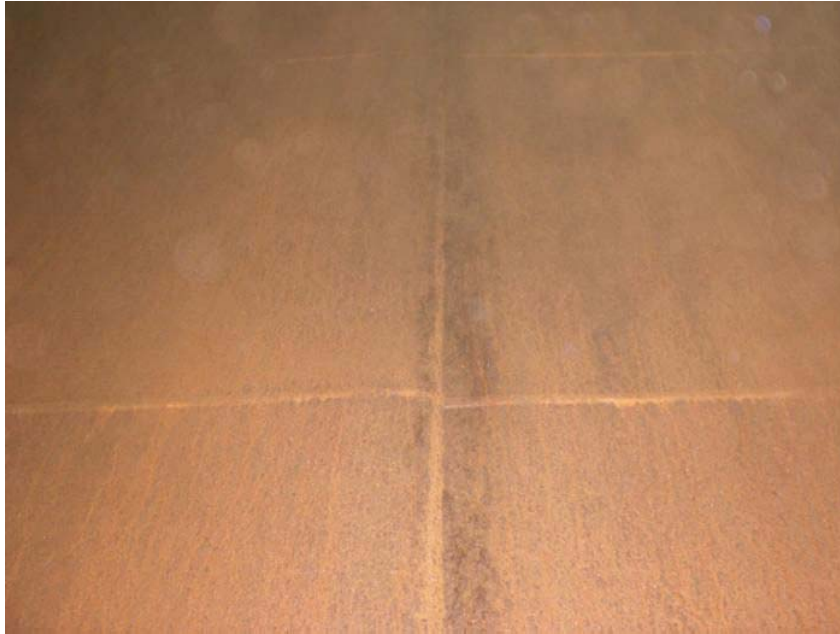
Pic 57: Vertical shell lap weld.
