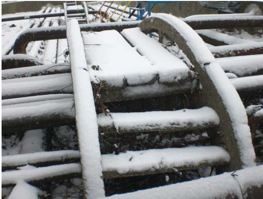
Pic 10: Misaligned concrete bridge. No handrail.
