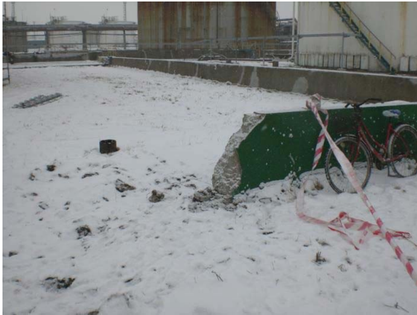
Pic 2: Broken dike wall.
