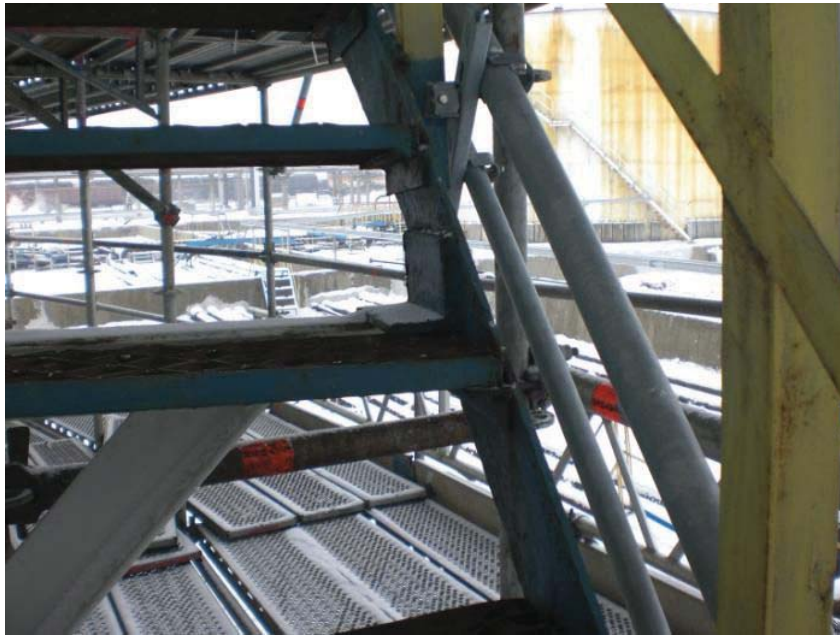
Pic 32: Spiral stairway in fair condition; minor paint failure and corrosion visible.
