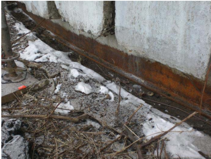
Pic 26: Damaged concrete ring, heavy vegetation. Soil under the tank bottom washed out.
