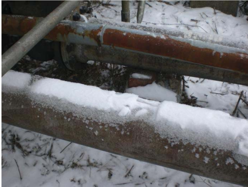
Pic 13: Pipe work lying on a concrete brick.
