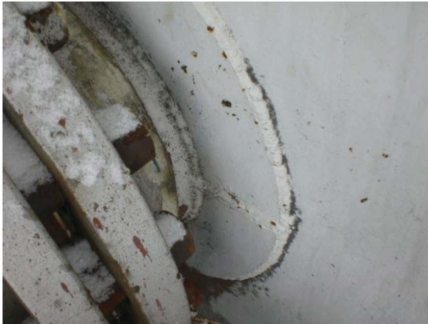
Pic 21: Reinforcement plate close up.
