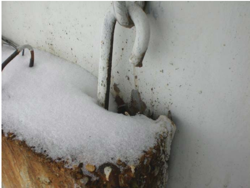
Pic 24: Concrete block connection. Paint failure and beginning corrosion on the shell plate.
