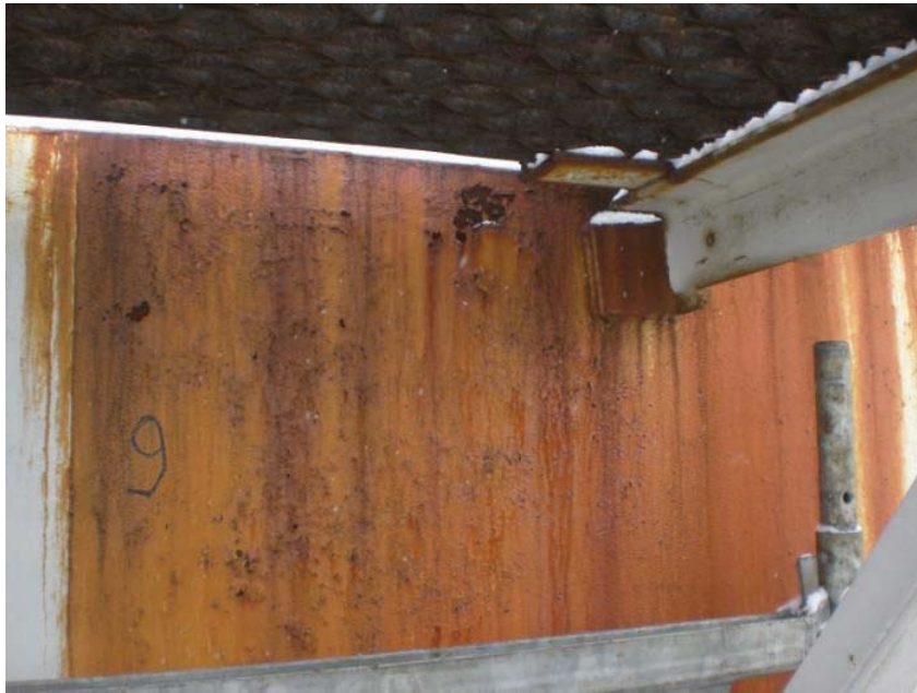
Pic 42: Paint failure and corrosion at the top of the shell.
