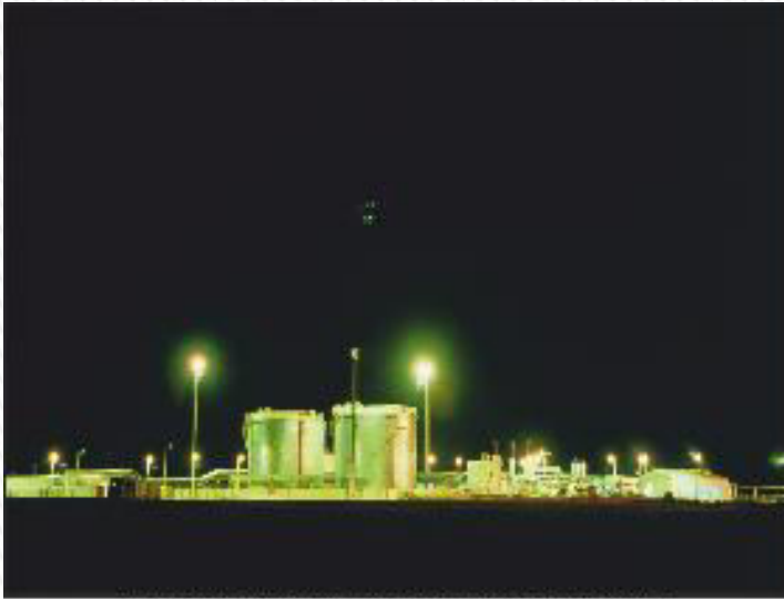
Tasbulat Separation Installation
