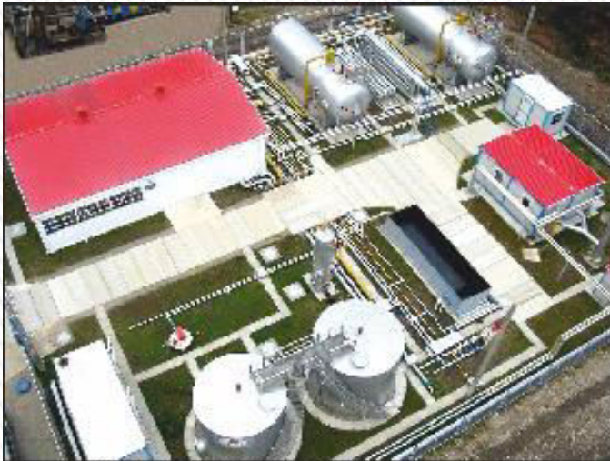
877 Mislea Separation Installation
