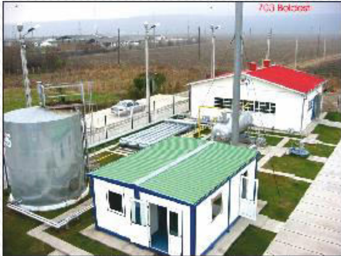
703 Boldesti Separation Installation
