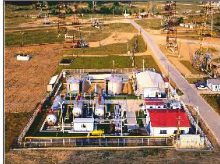
Ticleni Separation Installation
