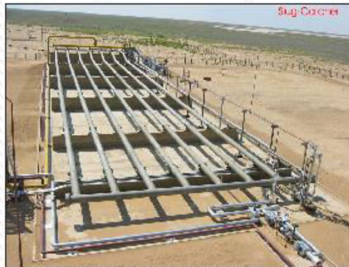
UKPG gas/condensate Separation Installation
