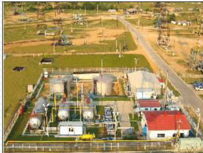
Ticleni Separation Installation
