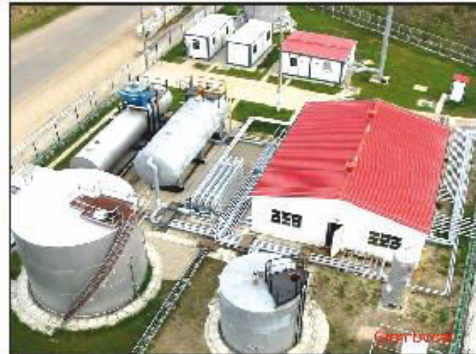
Glambocel Separation Installation
