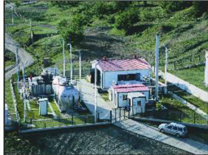
795 Lucacesti Separation Installation
