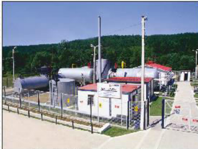
3 Balteni Separation Installation
