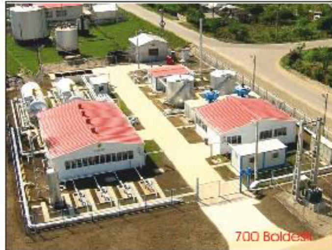
700 Boldesti Separation Installation
