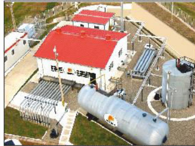
669 Boldesti Separation Installation
