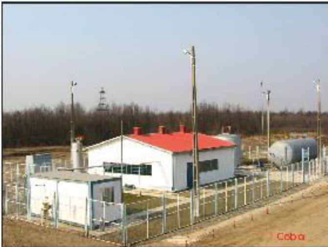
1 Cobia Separation Installation
