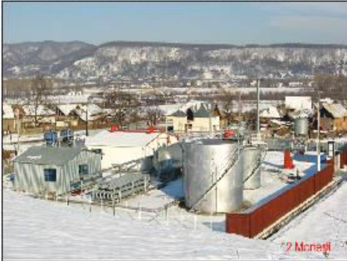
2 Manesti Separation Installation
