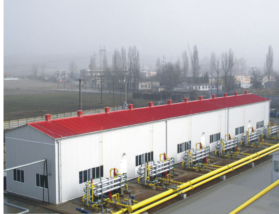
Ghercesti Electro-compressor Station
