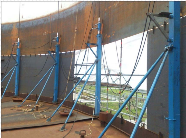
Tank supported on the floating deck
